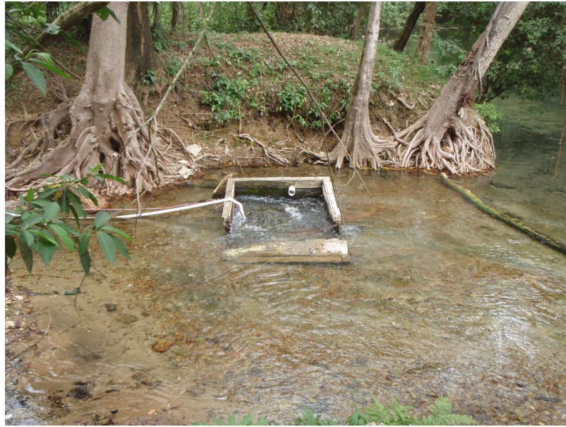
Figure 3. Water system source during the dry season. The solar pump is submersed in the spring.
