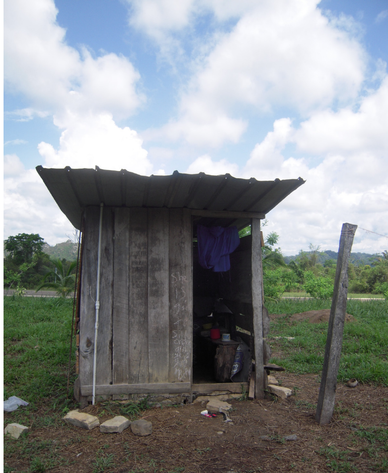
Figure 7. Typical water access point. Sheds are used to enclose the taps.
